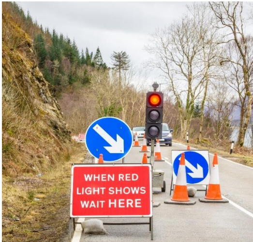
Temp traffic lights
